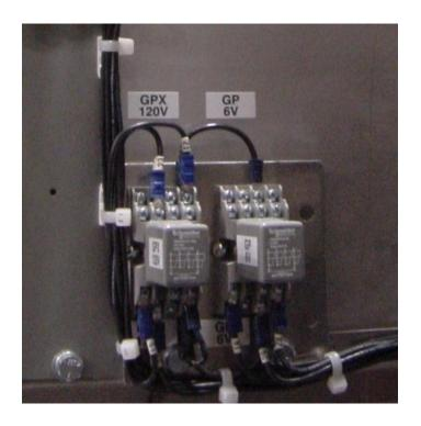
**OPERATION** GP and GCT are coordinated to sense approximately 10-amps primary ground current (zero-sequence). GP operates instantaneously when this ground current is sensed. As shown in the Schematic Diagram, GPX instantaneously seals-in to energize WIL and to open main contactor. Opening time for opening main contactor is the sum of operating times for GP, GPX, and main contactor. Opening times for Ground Faults of 10-12 amps or higher, are -
